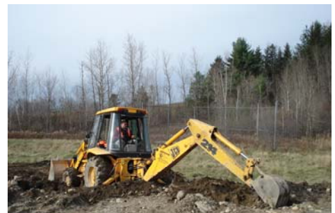
Forestry students gain excavation skills
